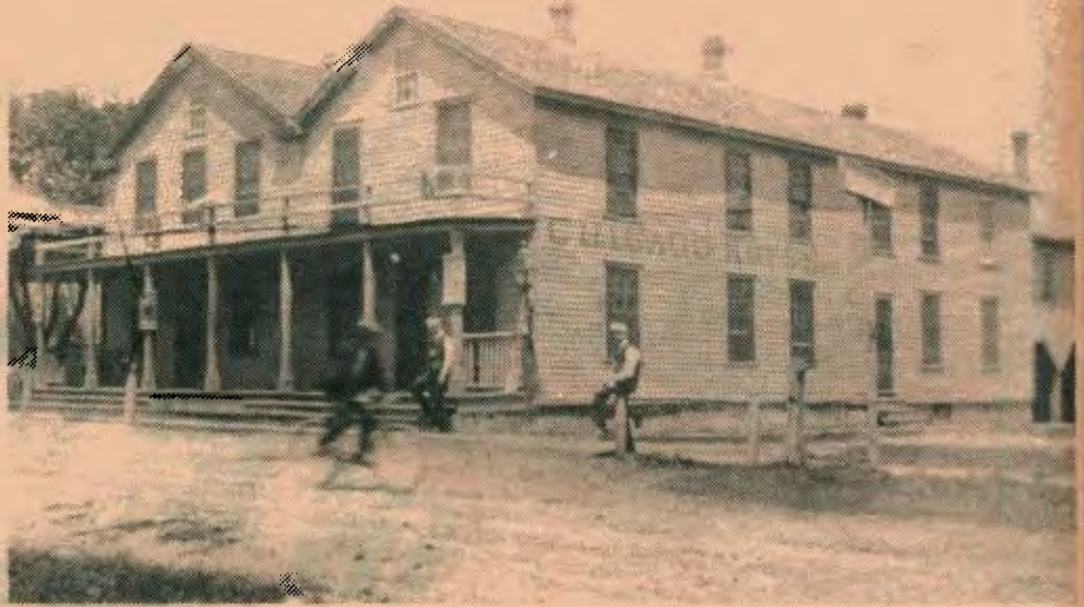
The Chicago House at 141 S. Milwaukee Ave. was built in 1873 by George Armbruster on the site now occupied by Hein's Pub.
